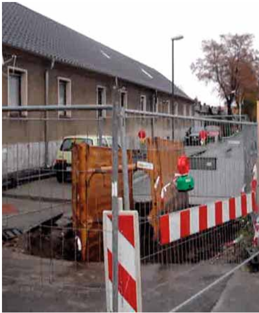
Baugrube in Zschornewitz
